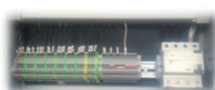
The machine has an electrical panel mounted inside of the main column.
